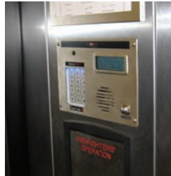
A reader/intercom unit can be installed within an elevator car.
