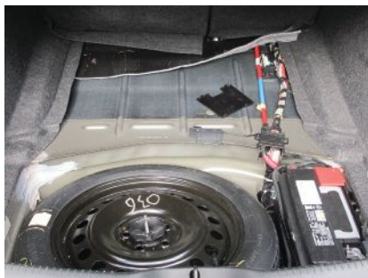
The junction box where I had to connect the Smart Pro was as far inside the trunk as you can get and under a flap of carpet.
